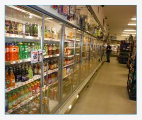
Doors on dairy cases and night curtains on meat and produce cases as well as new refrigeration controls, motors and LED case lighting at the Farmingdale Shop n Bag resulted in an estimated 30 percent reduction in energy use.
