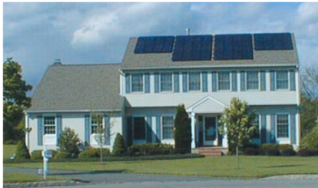
Residential pitched-roof installation in NJ
