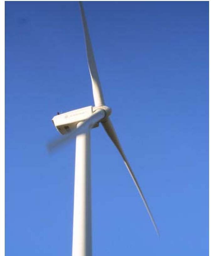
Photo courtesy National Renewable Energy Laboratory
