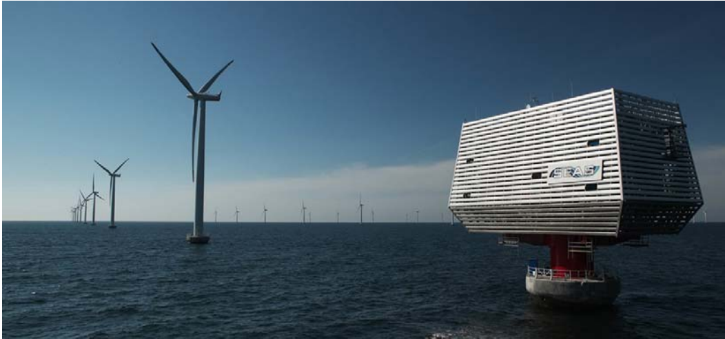
Figure 2.5: Nysted Offshore Substation and Wind Farm 13
