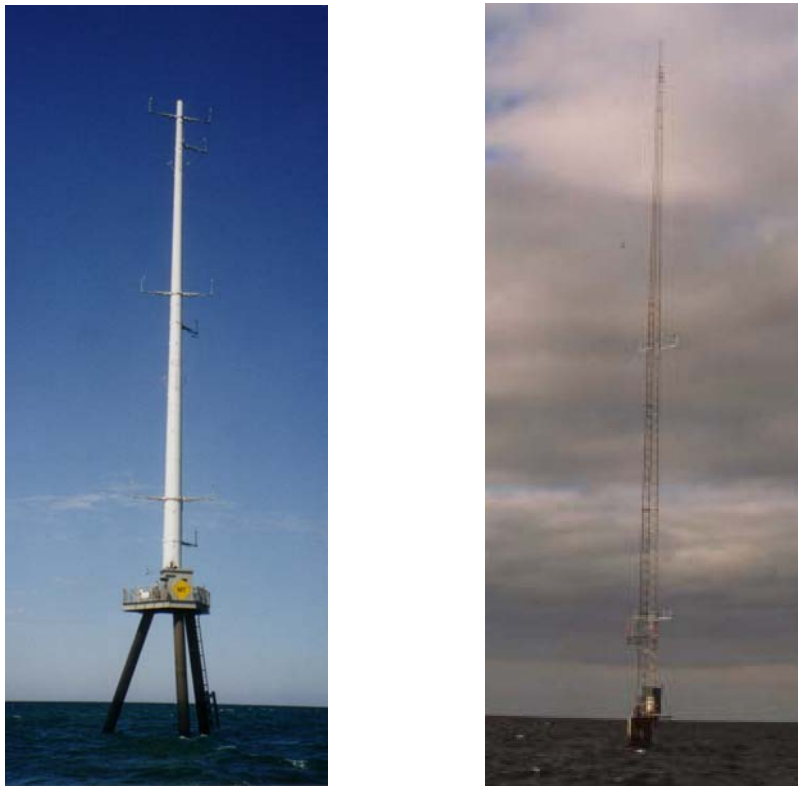
Figure 2.6: Cape Wind Meteorological mast (USA), Nysted Meteorological mast (Denmark) 14
