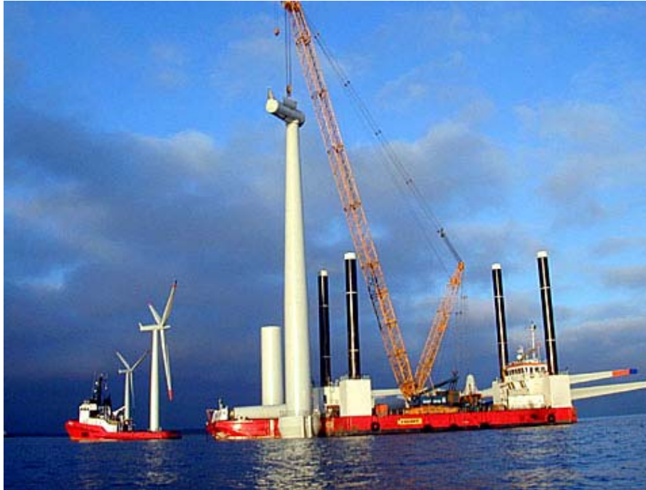
Figure 2.4: Installation Barge installing Bonus Turbine at Samsø, Denmark 12
