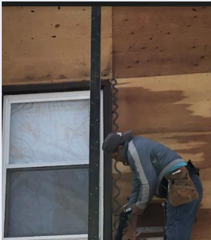
Liquid flashing application at window jamb
